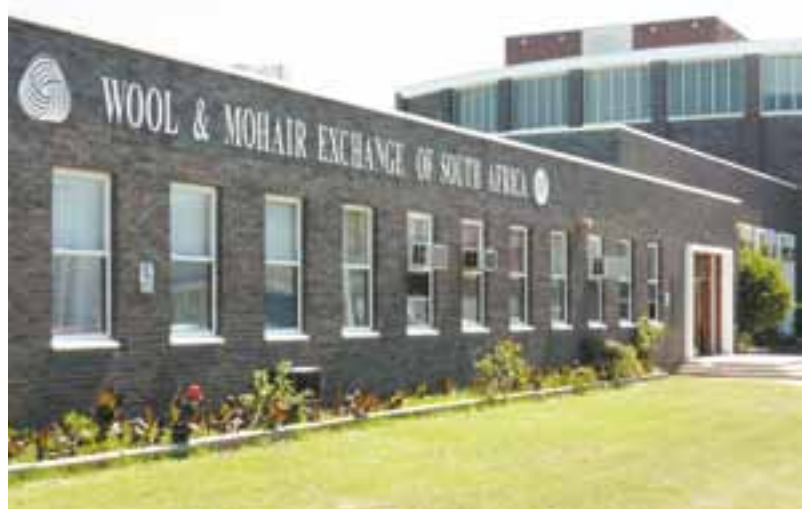
The Wool & Mohair Exchange building in Grahamstown Road, Port Elizabeth.
